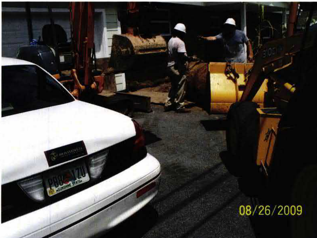
Picture 2: UST 1235Dove being removed.
